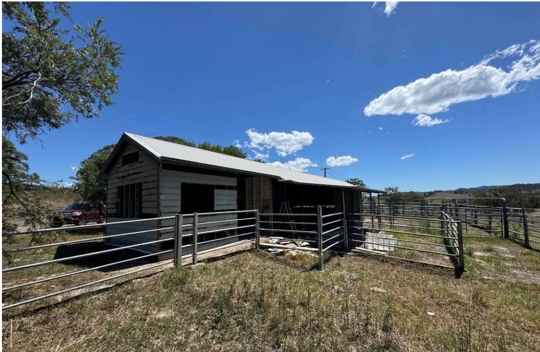
PHOTO 1 - EXISTING BUILDING LOOKING SOUTHWEST
